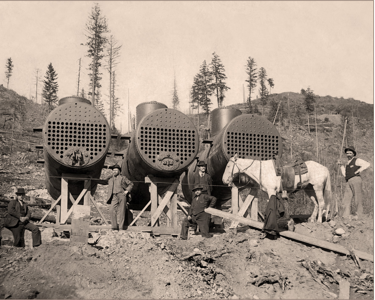
These giant compressors for the Le Roi Mine, were built by the Ingersoll Rock Drill Company, Montreal, and shipped by rail across Canada to Rossland. A Red Mountain Railroad spur line transported the heavy equipment to the entrance to the mine.
