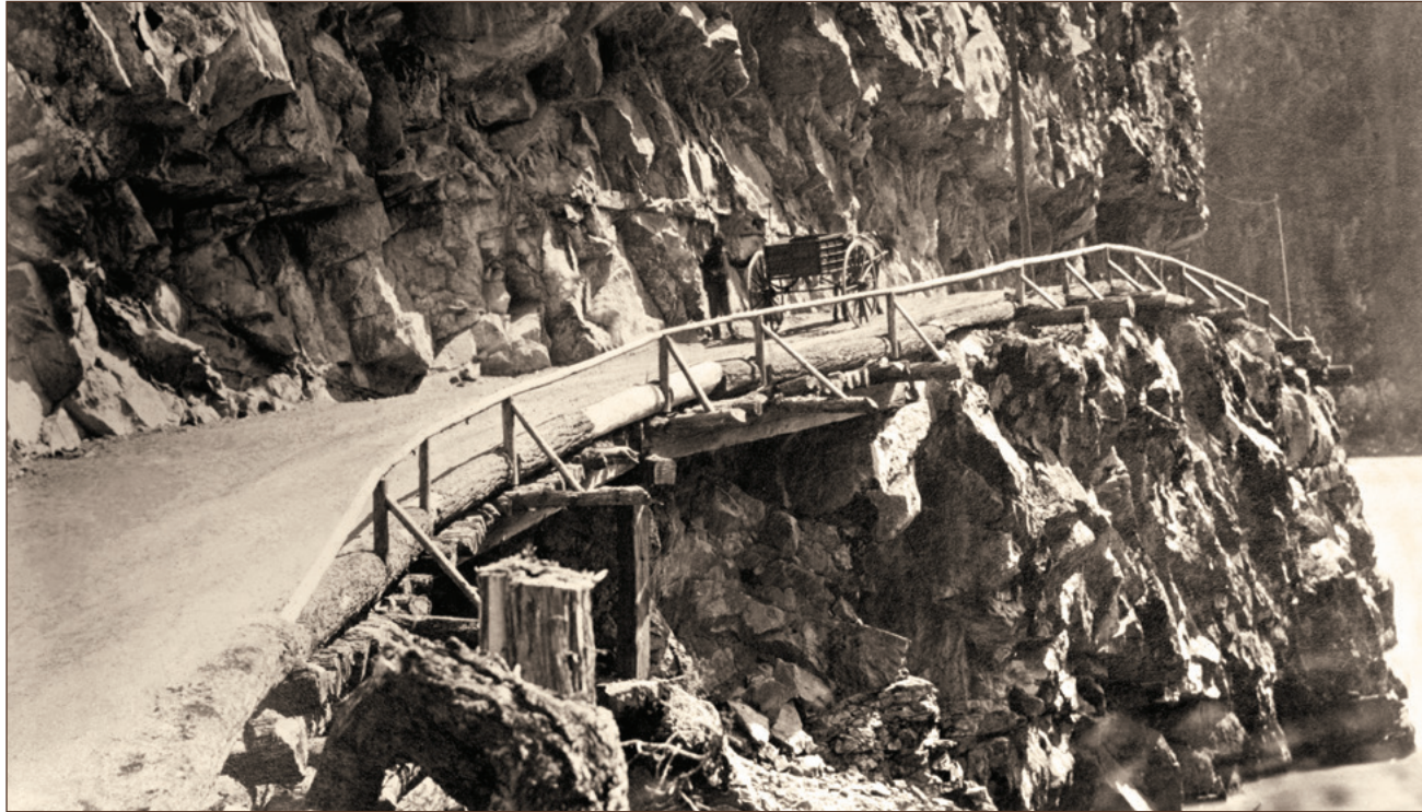
Chapman's Bar Bluff was part of the first 6 mile section of the Cariboo Wagon Road north of Yale that was built by the Royal Engineers between May and November 1862. The road had to be blasted from rock or suspended over the the many tributaries into the Fraser River on cribbing and bridges. Note photographer Dally's horse and buggy on the road.
