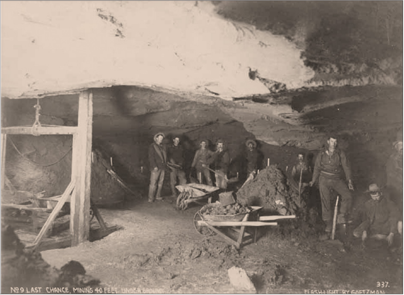
MINERS WORK THE LAST CHANCE CLAIM ON ELDORADO???BONANZA??? CREEK 40 FEET UNDERGROUND. THE MINERS HAVE MODIFIED A SHAFT INTO TWO COMPARTMENTS TO RAISE LOADS OF ORE ON WHEELBARROWS TO THE SURFACE . THIS REVOLUTIONARY INNOVATION ACCELERATED MINING ACTIVITY IN THE YUKON.
