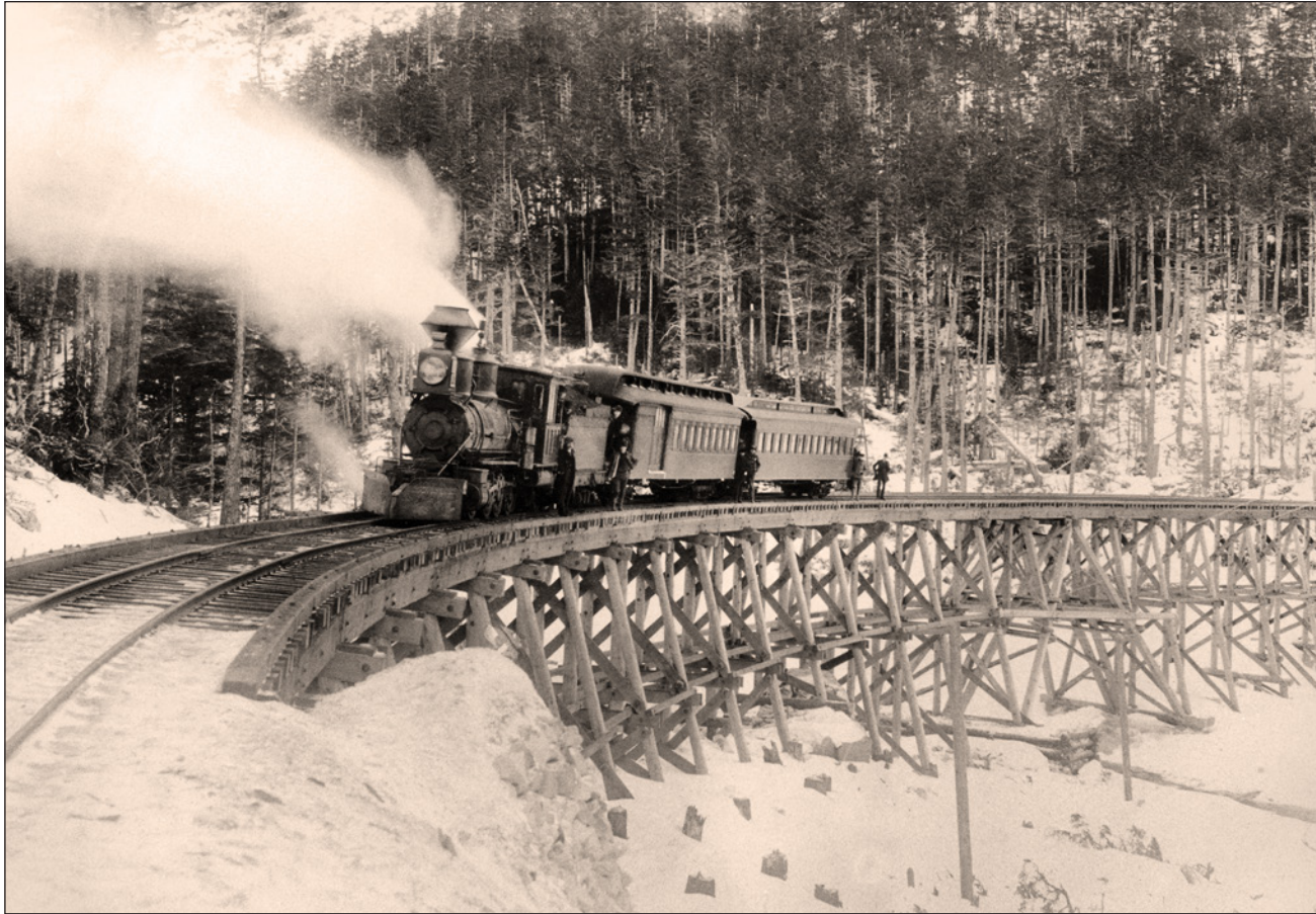
CROSSING THE EAST FORK OF THE SKAGUAY RIVER The first passenger train over the White Pass and Yukon Railway crossing the east fork of the Skagway River en route to the summit of White Pass, Alaska, 20 February 1899 UNIVERSITY OF WASHINGTON DIGITAL ARCHIVES HEG659 PHOTOGRAPHY BY ERIC A. HEGG
